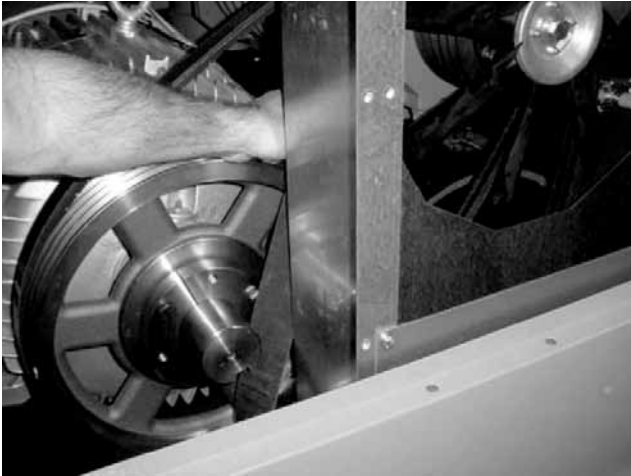
(5) Pass the belt between the sheave and the exhaust plenum.
